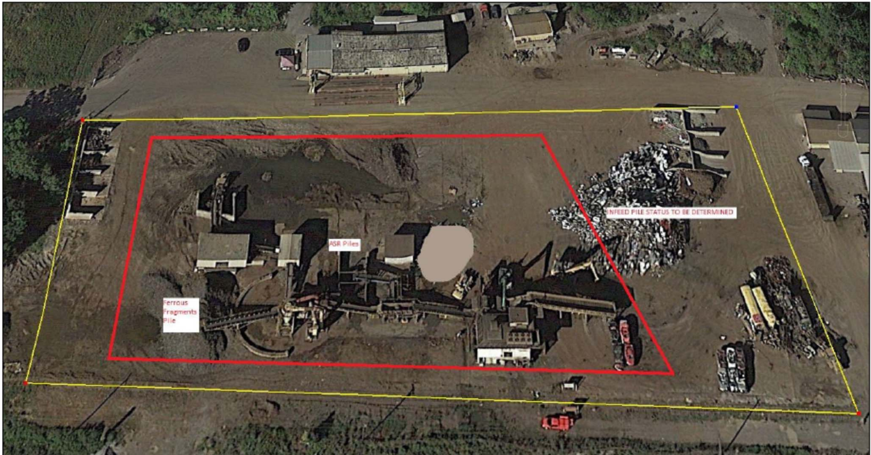
Figure 3: Satellite View of PSC Metals – Beaver Falls Shredder Yard (Yellow box indicates estimated Class 1 extent; Red indicates Remedial Decontamination and Waste Removal)
